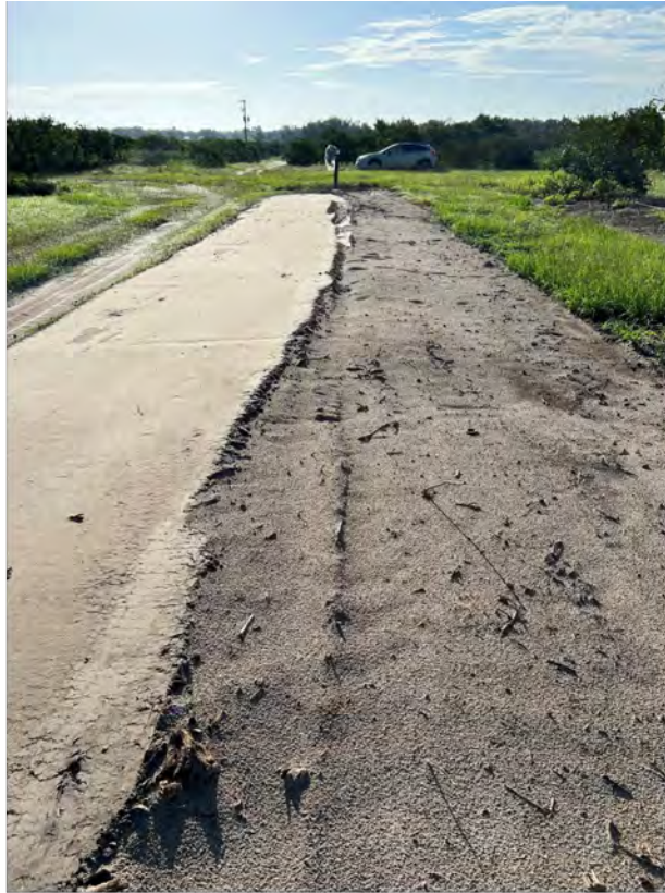
One pass of roller on the rotovated bed
