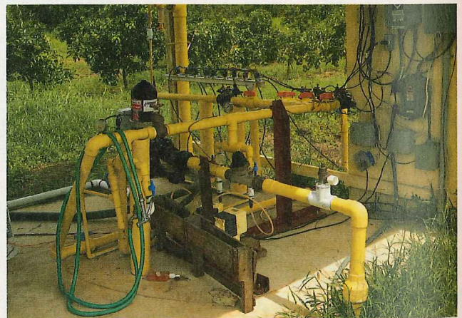
Open hydroponic systems are designed to increase productivity by continuously applying a balanced nutrient mixture through the irrigation system.
