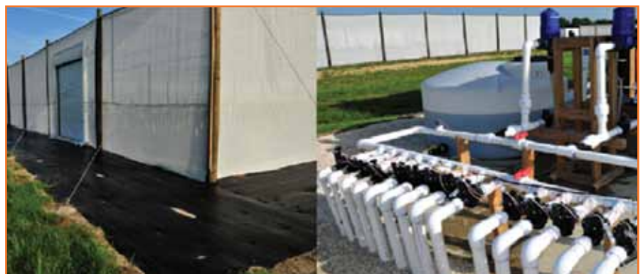
Figure 1. Left: A pole-and-cable, anti-insect screen house at the UF-IRREC in Fort Pierce. Right: Irrigation/fertigation valve manifold with liquid chemical proportional injectors in the upper right-hand corner of the image.
