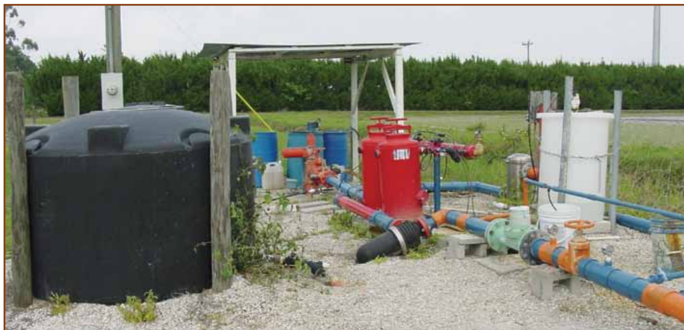
Figure 3. Fertigation system including backflow prevention devices.
