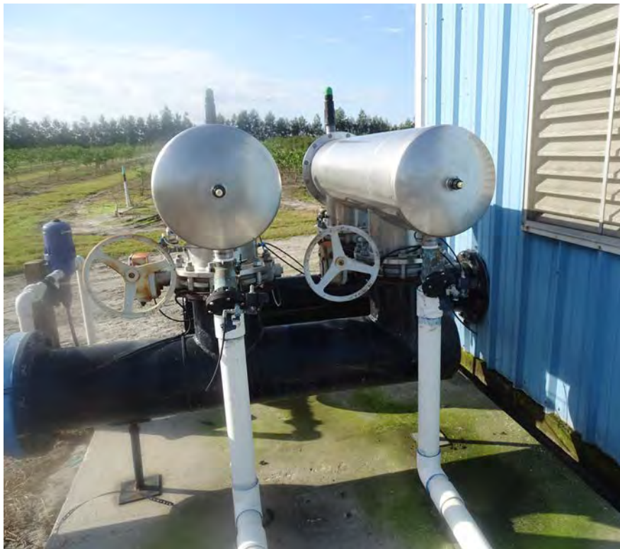
Figure 2. A screen filtration system is used with microsprinkler irrigation and fertigation.
