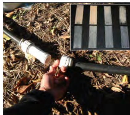
Figure 1. A 3/4-inch PVC coupling found in plumbing-supply stores serves well as an in-line glass slide holder. Observing the amount, type and rate of scale deposition occurring on a clean side (inset) can help determine the scaling potential of the irrigation water and the effect of injected scale-inhibiting chemicals. (Source: Obreza et al., 2017)
