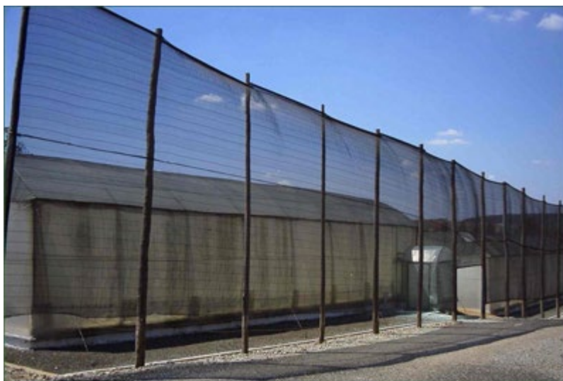
Fig. 1. A greenhouse nursery with an artificial windbreak in place for canker management
